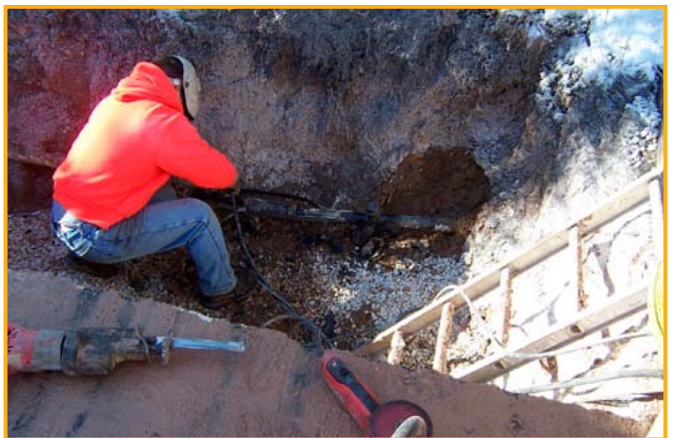
Gas company repairing damaged 2 inch steel main.
